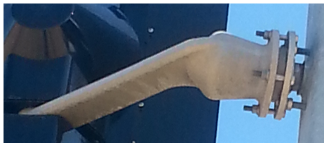
THREADED HUB AND FLANGE POLE ADAPTOR
