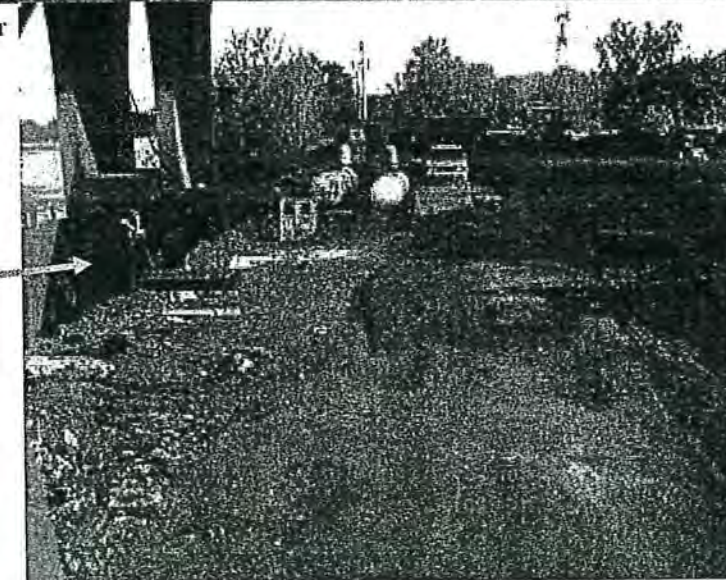
Priming or washing out of pumper truck into empty concrete truck for total containment of washout slurry.
