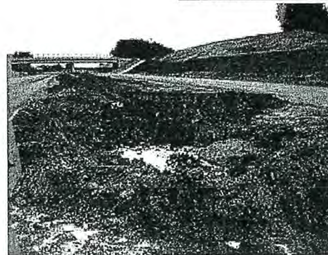
High cohesive, low infiltration soil berm
