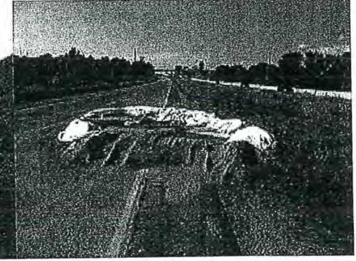
Mixing sand berm with plastic liner
