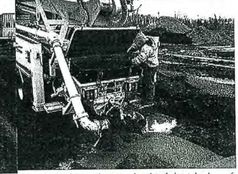
Final remnant of pumper hopper washout into designated and signed washout trap.
