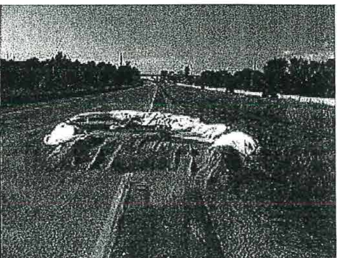
Mixing sand berm with plastic liner
