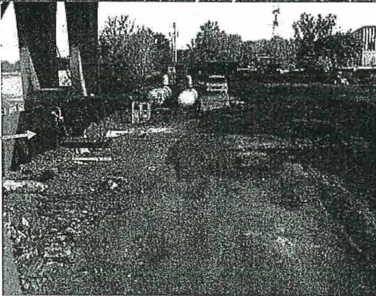
Priming or washing out of pumper truck into empty concrete truck for total containment of washout slurry.
