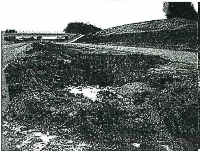
High cohesive, low infiltration soil berm
