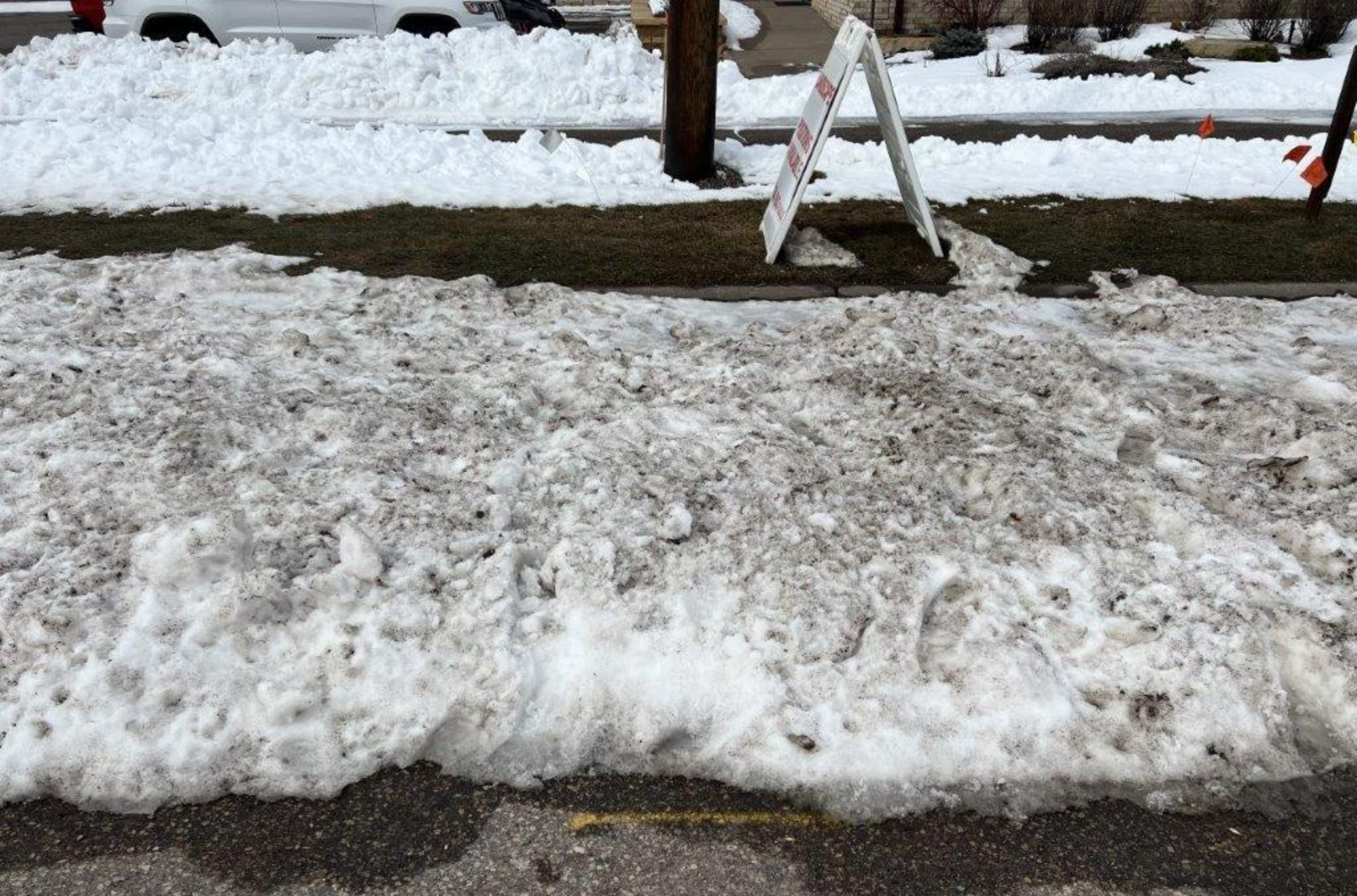
New pothole location (facing WB - curb)
