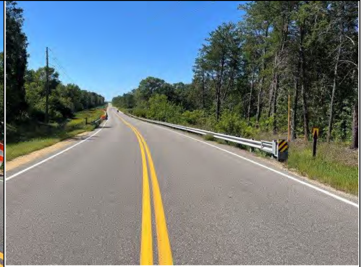
Photo 2 – View of Bridge 02502 looking to the west along CSAH 28.
