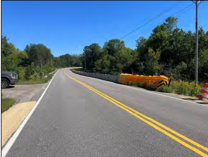
Photo 1 – View of Bridge 02502 looking to the east along CSAH 28.
