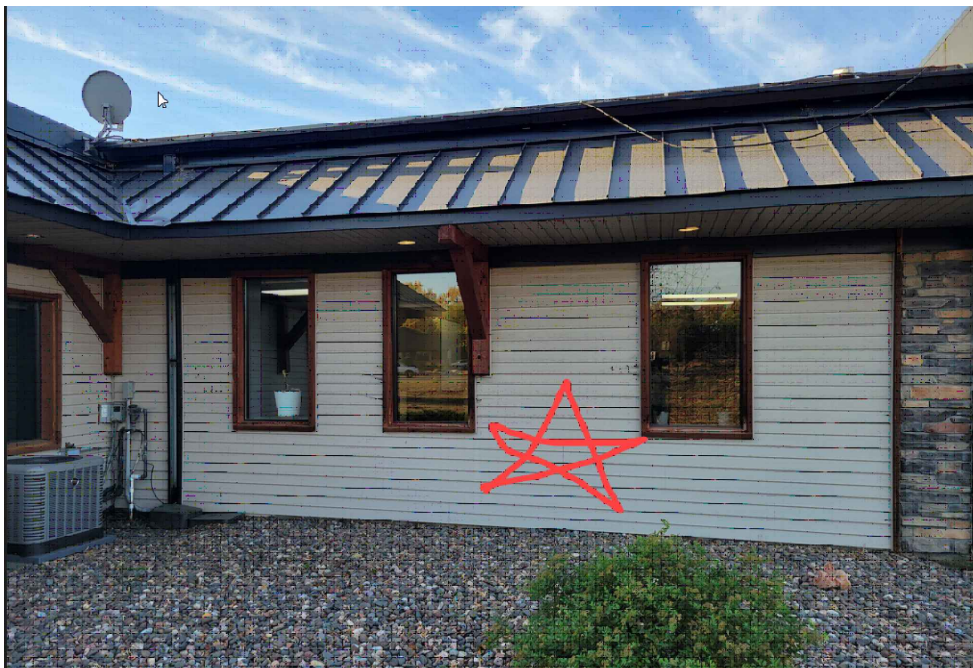
NEW METER LOCATION
